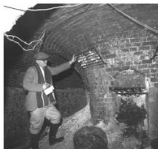
4. Inside the Gilman Road lime kiln, 1971, showing circular access tunnel and central firing pot with extraction chute. The investigator is the chalk geologist Norman Peake.
