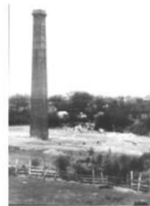
3. The brick kiln at Hooper Lane was demolished in 1950s.
