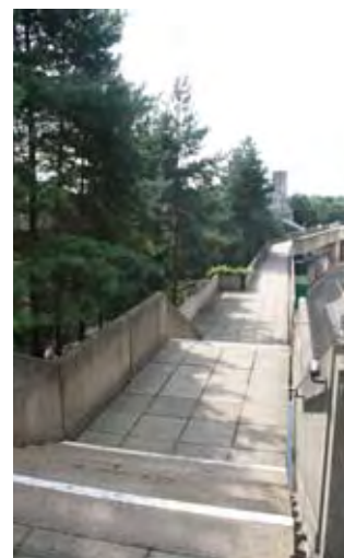
Above: Part of Lasdun’s original walkways.
