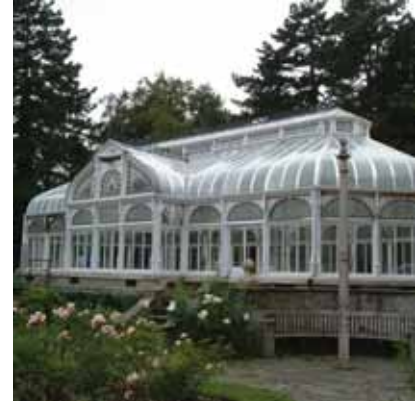
Fig 35: Carrow House Conservatory and decorative pole for sunshade
