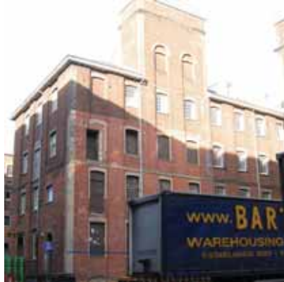
Fig 20: Late 19th century building at Carrow Works
