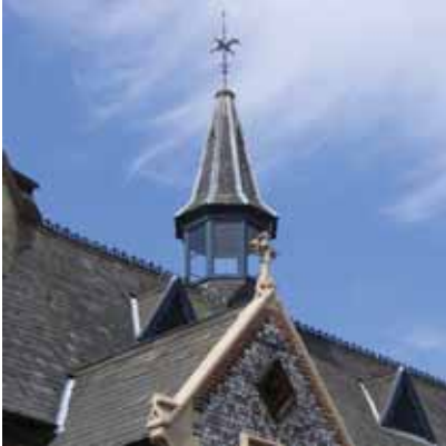
Fig 36: Ornamentation and knapped flintwork at the school on Carrow Hill
