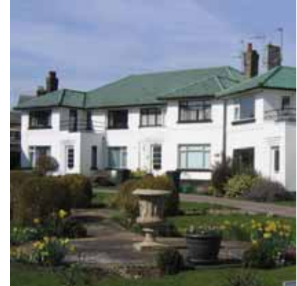
Fig 24: Bracondale Court (1930s) is arranged around a 'green'
