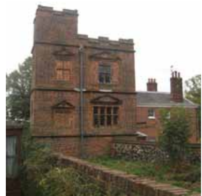
Fig 29: The tower to the rear of 58 Bracondale
