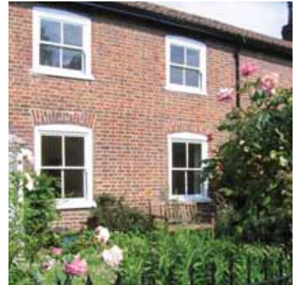
Fig 12: Terraced housing on Ice House Lane (c. 1830) with small front gardens defined by cast-iron railings and with a pedestrian alley providing access
