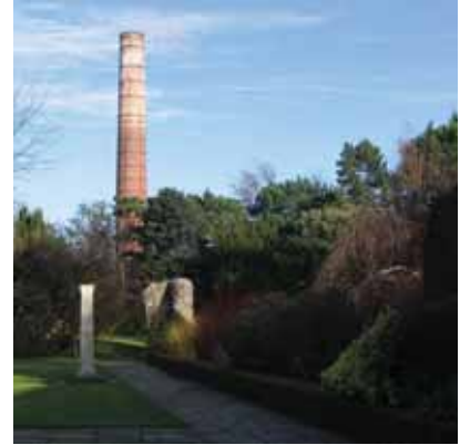
Fig 18: Carrow Works chimney viewed from Carrow Abbey
