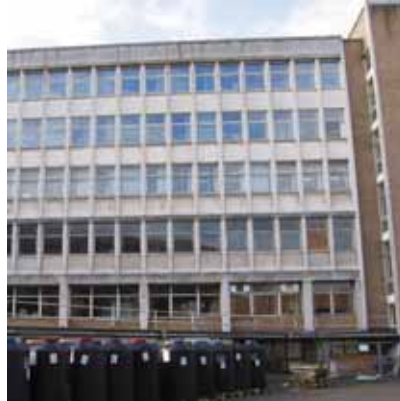
Fig 23: The north-east elevation of the Carrow House extension
