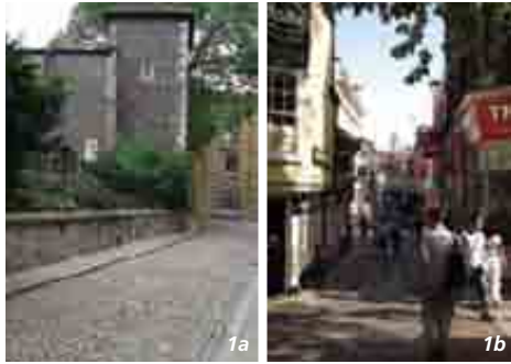
1. Flint cobble carriageway, granite kerb St Andrew's Hall Plain, Yorkstone paving 1b. Relaid setts and drainage channel Lobster Lane
