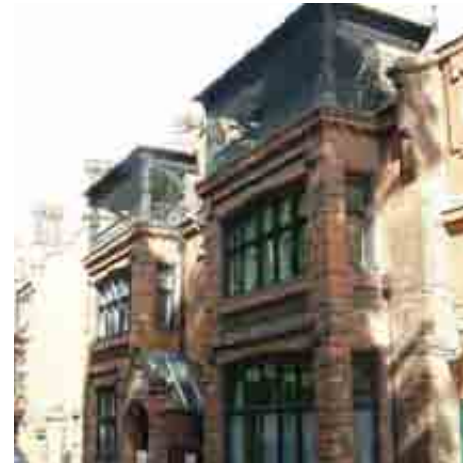
C19 Villas Chapel Field North
