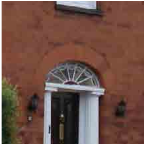
Red brick (gauged) House on Sussex Street
