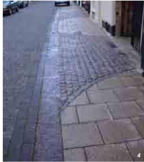
4. Relaid granite setts and kerb Kings Street
