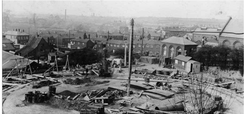
Construction of gas holder. Photograph ©Norfolk County Council
