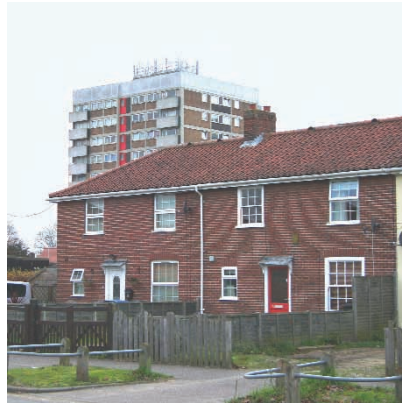
A group of three 1960s blocks of flats dominate views out of the conservation area to the west
