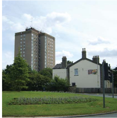
Winchester Tower – a modern landmark adjacent to the conservation area.
