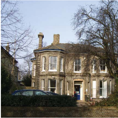
Retaining existing walls and landscaping helps to screen parked cars in street views.
