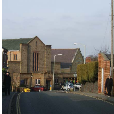
St Peter's Methodist Chapel is an important landmark at the junction of five streets.
